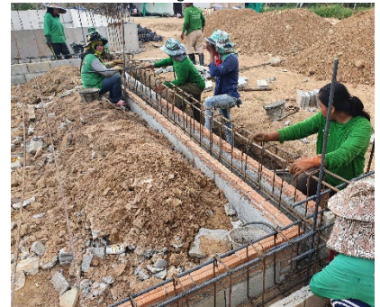
Sub-ground beams
