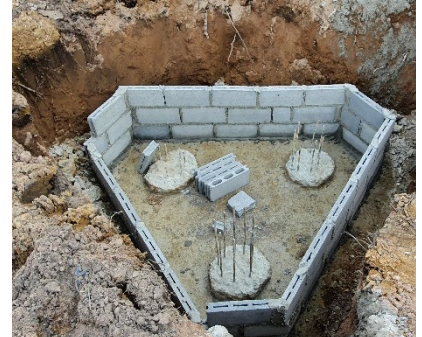
Footing formwork
