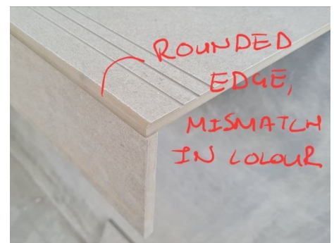
Half Bull Nose Tile Edge, Mismatch in edge colour
