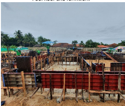
Ground floor beams (raised above ground)
