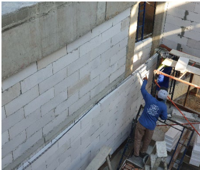
Q-Con Cavity Walls
