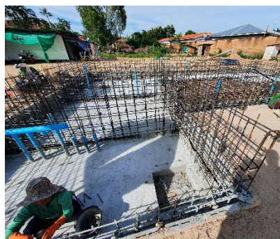
Pool walls & overflow tanks (under ground)
