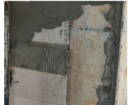
Steel wire mesh reinforcing for plaster
