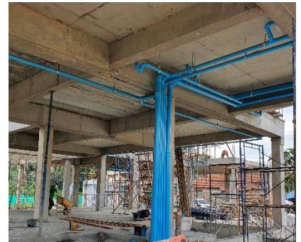
Plumbing 1 st fix
