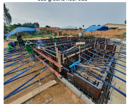
Swimming pool shuttering
