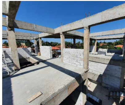
Floors, Beams & Columns completed
