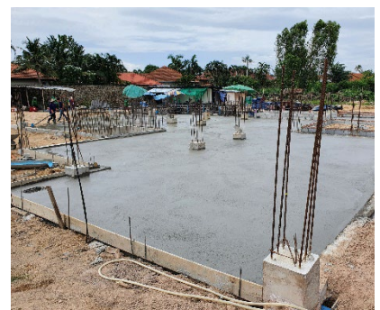
Sub-ground floor slab
