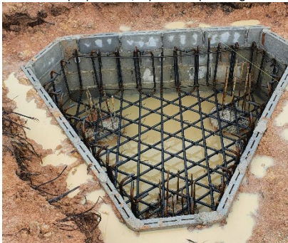
Piles and Footing "F3"
