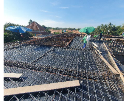
2 nd floor structure beams & floors
