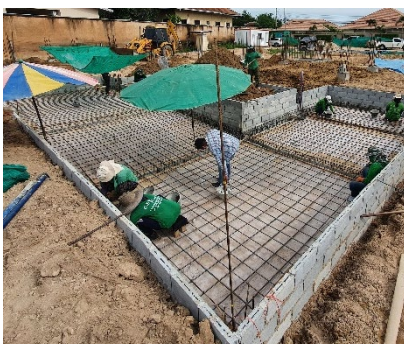
Pool floor and formwork
