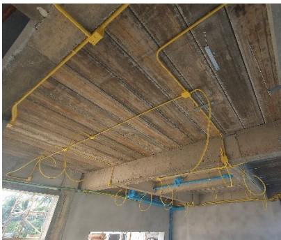
Electrical 1 st Fix, (Require switch, socket & lighting positions)
