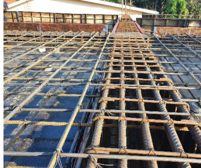
Rebar work for beams and floor slabs
