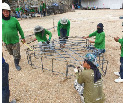
Rebar work for footings
