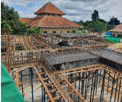
2 nd Floor Shuttering
