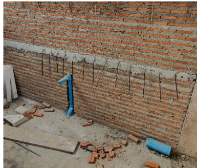
Reinforced lintel for countertop, Plumbing 1 st Fix.
